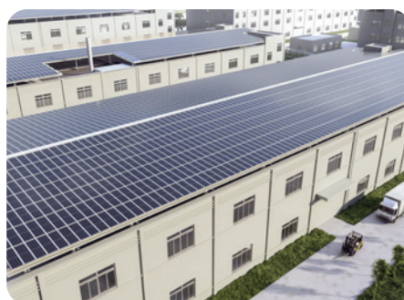
Flat-to-pitched Roof Conversion
